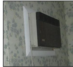
Cooling is provided by individual room air conditioners that are primarily installed through exterior walls, or in some cases in the lower sash of double hung windows.
