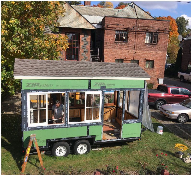
Photo caption: Blue Moon Builders installed custom-made sliding windows on the Cure Porch on Wheels in October. Courtesy of Historic Saranac Lake.
